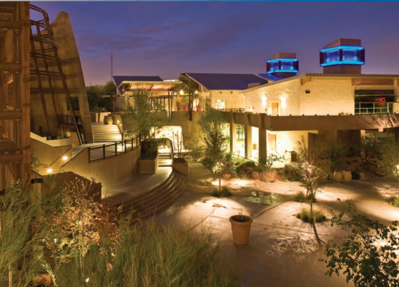
Las Vegas Springs Preserve, Las Vegas, NV. Owner: Las Vegas Water District. Architect: Tate Snyder Kimsey Architects, Poggmeyer Design Group and C+B Nevada. General Contractors: J.A. Tiberti Construction and Whiting-Turner Construction Co.
